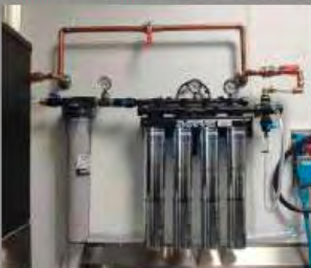
Pentair Configuration I – Base Filtration
